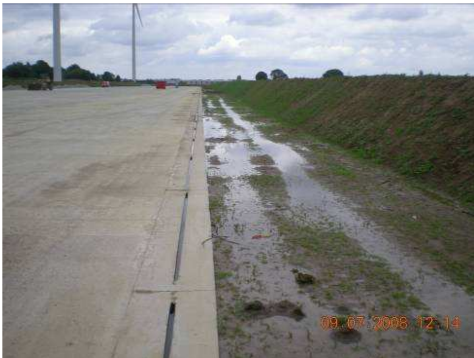
FOTO PLATFORM + AFWATERINGSGOOT
