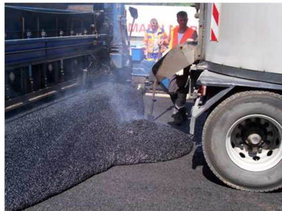
Frankfurt: 2007: A3 – Lage Temp GA met 20/30 PX – 230°C (traditioneel 270°C)
